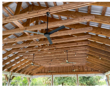
Improved electric and addition of new fans under the pavilion
