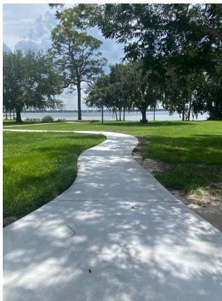
New sidewalks leading to the Indian River Lagoon
