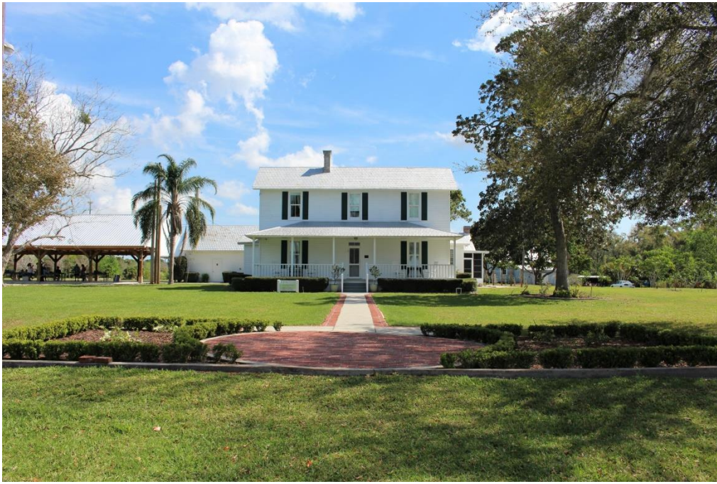
HISTORIC 19 TH CENTURY WATERFRONT HOMESTEAD, GROVE AND FARM ON THE INDIAN RIVER
